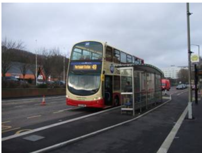
Cycle Lanes on the inside of bus stops along the Lewes Road Corridor, Brighton
