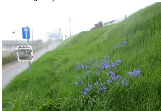
Basin Road North embankment
