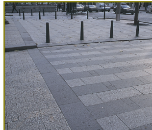
Remove ALL guard railing - use bollards instead if necessary. Champs-Élysées, Paris, France
