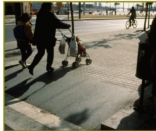
Ramp at street intersection that ensures that wheelchair users and people with prams may move around freely. Barcelona, Spain
