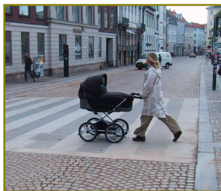
Crossings integrated with the pavements contribute to the visual quality while maintaining a consistent level for prams and wheelchairs. Copenhagen, Denmark
