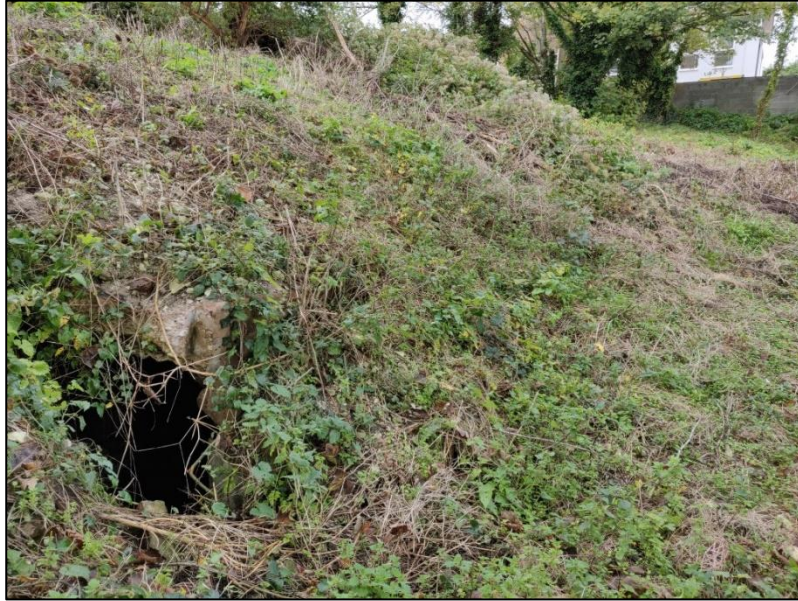
Photo 4.5 World War II air raid shelter in north-west of site
